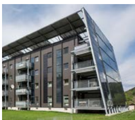
Retrofitting multi-family house Kapfenberg (AT)
